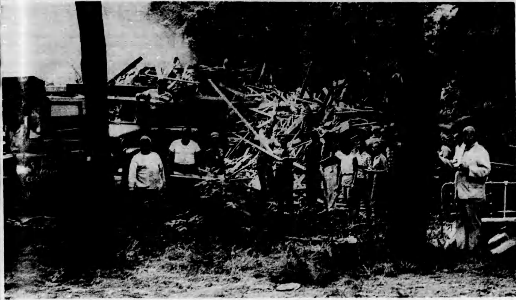
DO IT YOURSELF VERSUS URBAN RENEWAL —Volunteers engage in demolishing seven cottages in Beck-Wainwright area in step toward improving blighted condition as opposed to urban renewal plan. Councilman Don Fendler at far right supervised the work. (Al Porto Photo)
